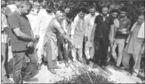
DDC member, Suresh Sharma starting road work at Akhnoor.
