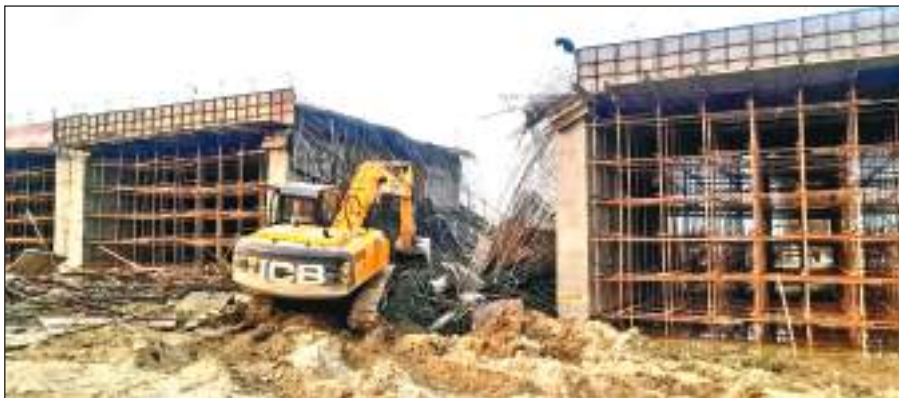
Shuttering of under-construction bridge over Devak River at village Koulpur Ramgarh collapsed.
