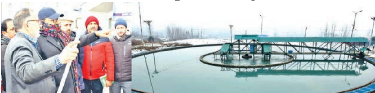
Minister for Jal Shakti, Javed Ahmed Rana inspecting on Water Treatment Plant Rangil in Ganderbal.
