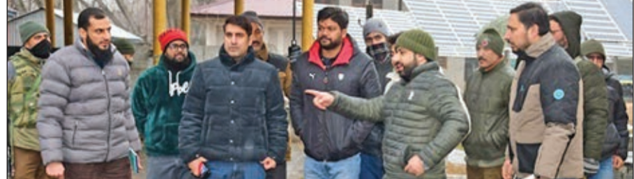
Secretary RDD & PR, Aijaz Asad visiting construction site of Yatri Niwas at Mata Kheer Bhawani Temple.
