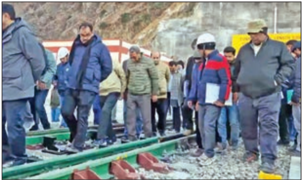
RSC Northern Circle Dinesh Chand Deshwal during statutory inspection of track.
