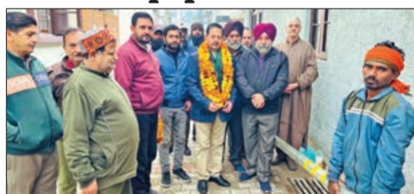
Former Dy Mayor Jammu Baldev Singh Billawaria inaugurating drinking water pipeline work in Gangyal.
