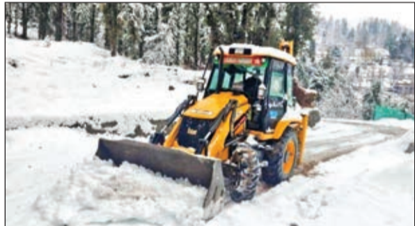
JCB engaged in snow clearance work on Jammu-Srinagar Highway at Ramban.
