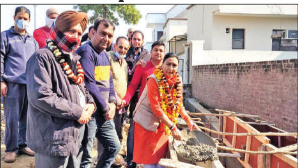
Councilor Ward-69, Gurmeet Kour Randhawa starting deep-drain work at Sainik Colony.
