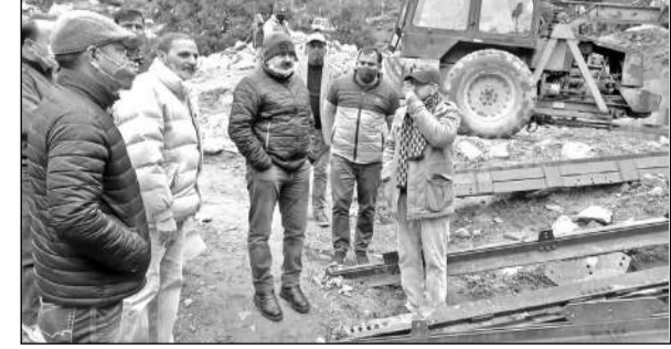
DC Kishtwar Ashok inspecting ongoing works.
