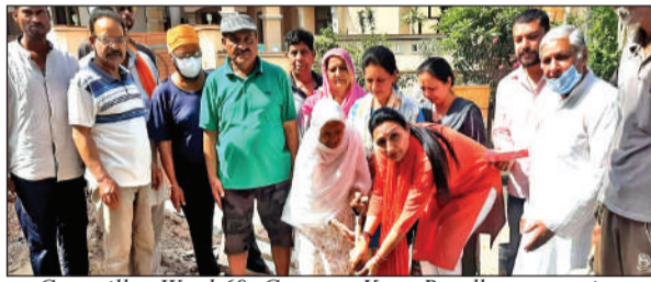
Councillor Ward 69, Gurmeet Kour Randhawa starting lane-drain work.
