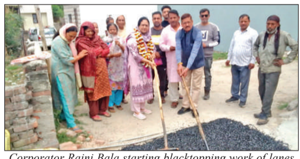
Corporator Rajni Bala starting blacktopping work of lanes in Ward 60.
