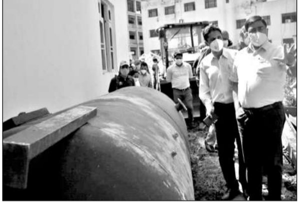
DC Rajouri, Rajesh K Shavan taking stock of work progress on oxygen concentrator plant.
