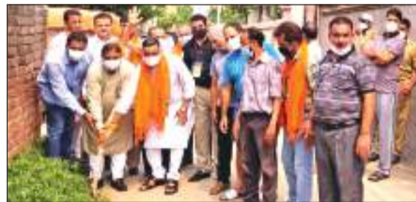
Former President BJP J&K Sat Sharma along with Corporator Sanjay Baru starting drain work.
