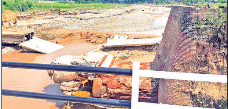
Duct of canal completely washed away depriving villagers of irrigation facility.
