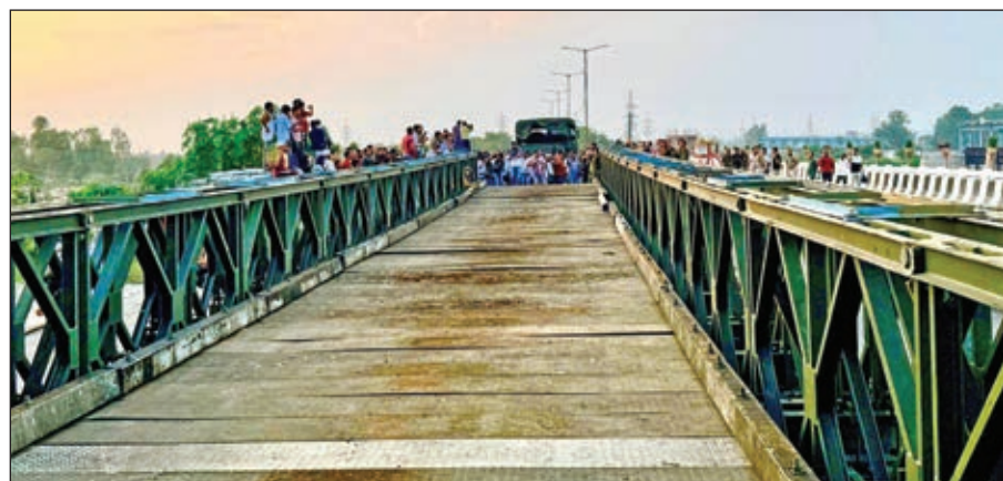
110-foot Bailey bridge constructed by army connecting flood-hit Tawi bridge. (Pic by Ashok Anand)
